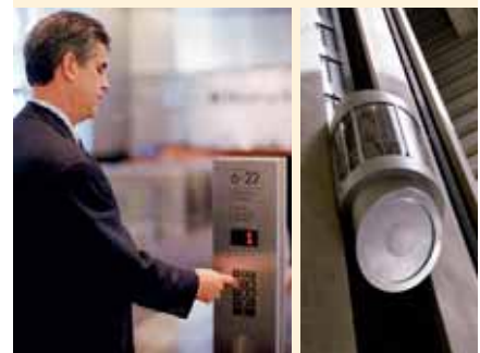
The Miconic 10 keypad resembles a telephone keypad (left). All-new elevator cabs (right) were part of the retrofit. Photos: Schindler Elevator Corporation
