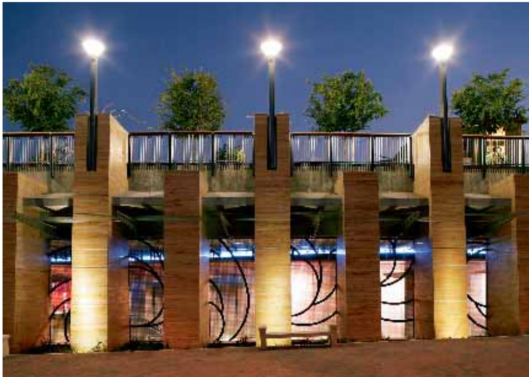
Gold travertine covers the meter-thick pillars, which are topped off with planters and decorative light fixtures. A trellis hangs above the window openings, which are filled with curving decorative metal forms and a barely perceptible bird netting.
