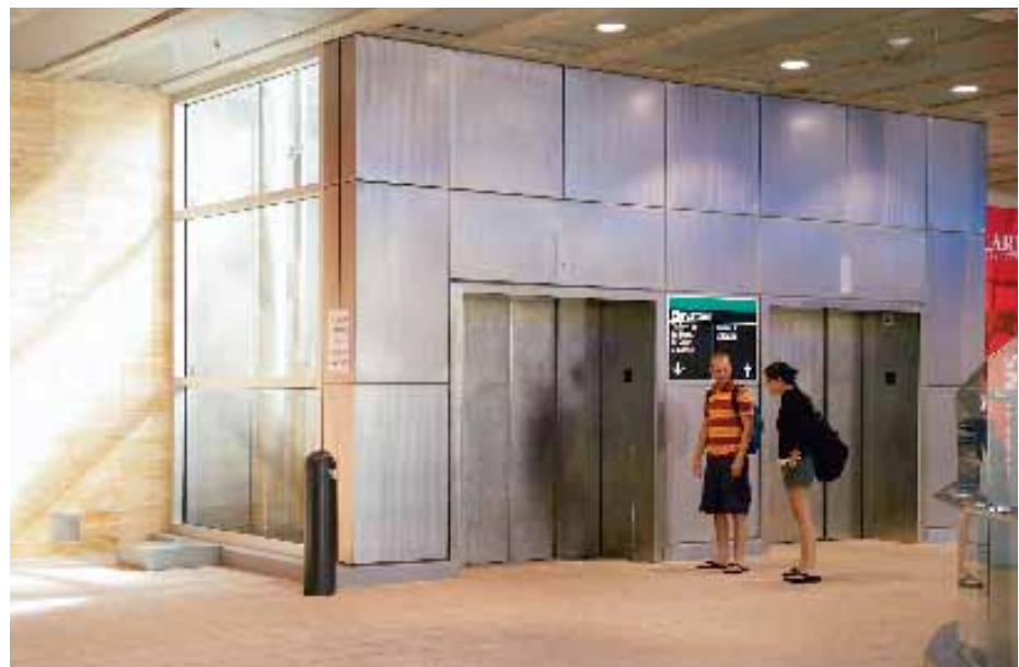
The elevator shafts have glass sidewalls that bring natural light from the street level to the mezzanine level (shown here) and to the pedestrian platforms below.
