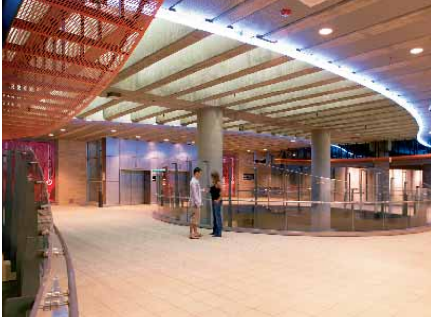
A blue cold cathode light tube streaks across the mezzanine ceiling. Acoustic insulation fills the caps between the concrete ceiling beams, and is also hidden behind the orange-red perforated metal ceiling panels.
