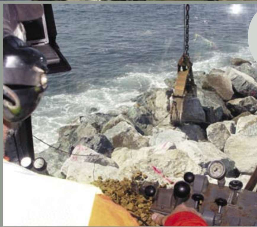
Crane operator Bill Pankey carefully places a stone on the jetty.
