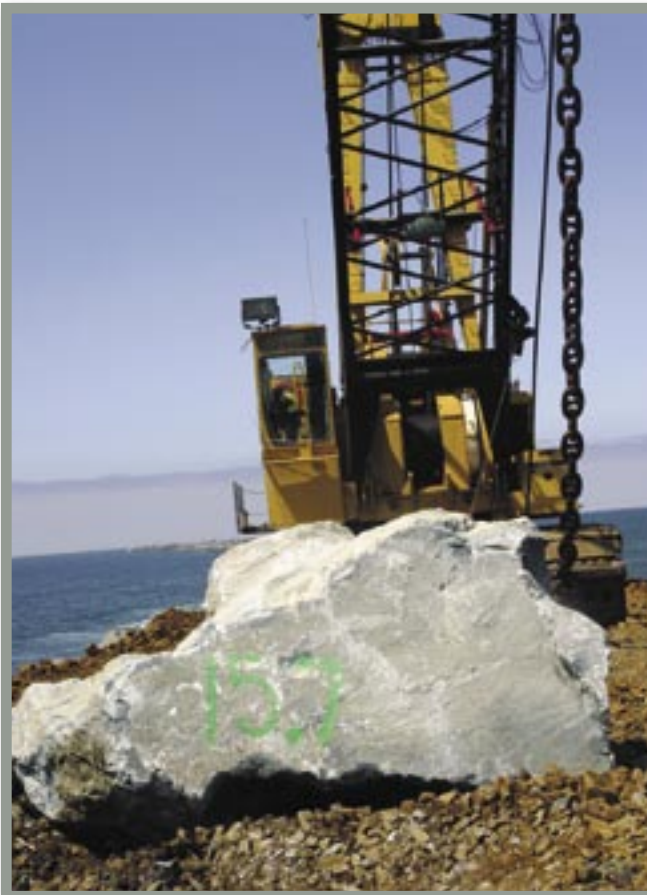
Kiewit Pacific's Manitowoc 4600 Vicon crane prepares to pick a 15.7-ton rock.
